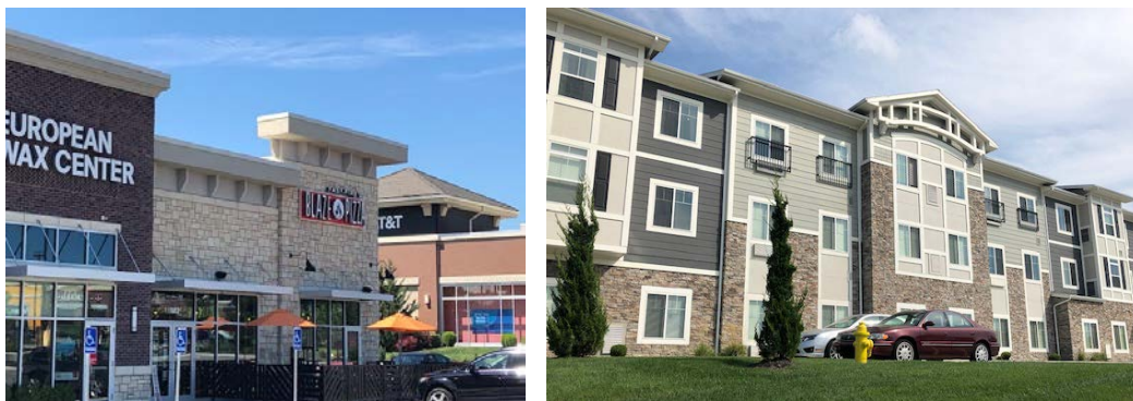
Example of appropriate use of façade expression
