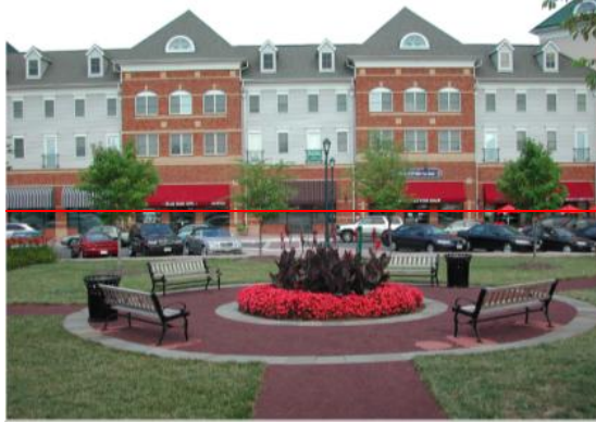
Figure 2. Class C design with buildings facing a square. Civic spaces are allowed, but not required, in TOD.
